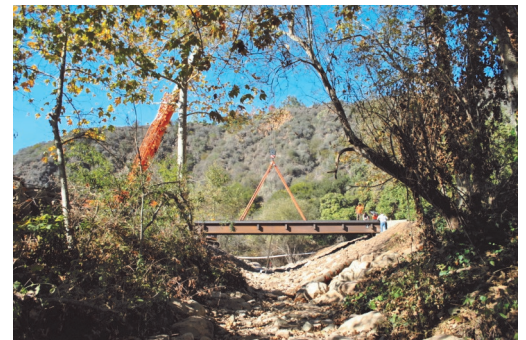
FROM UPSTREAM LOOKING BACK DOWNSTREAM SHOWS THE CRANE INSTALLING THE NEW BRIDGE ACROSS THE CREEK.
