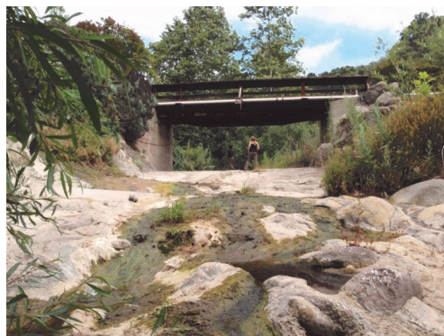
A BEFORE PHOTO OF THE PROJECT SHOWS THE LARGE AND STEEP SECTION OF CONCRETED CHANNEL AND THE UNDERSIZED BRIDGE THAT WERE REMOVED TO PROVIDE FISH PASSAGE THROUGH THE SITE.
