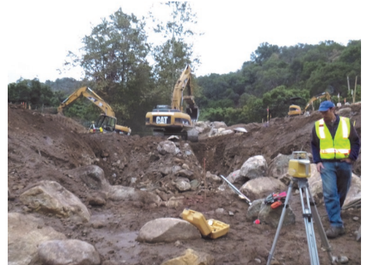
FROM THE DOWNSTREAM END LOOKING UPSTREAM SHOWS THE CONSTRUCTION OF THE NEW STREAM CHANNEL.
